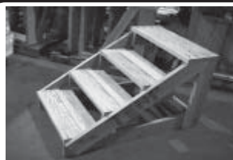
200040 Temporary Wooden Steps
